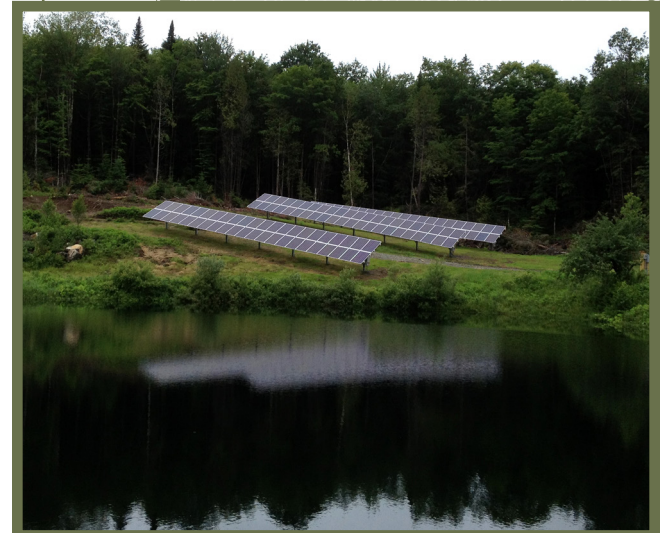
A solar panel array at the Bald Hill Fish Culture Station is supplementing approximately 75% of the facility's electrical demand.
